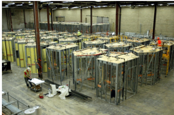
Miami Valley Hospital Southeast Addition Modular Construction, Skanska
