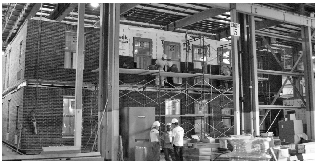
Fig. 1. Module production of a 3-story dormitory project
